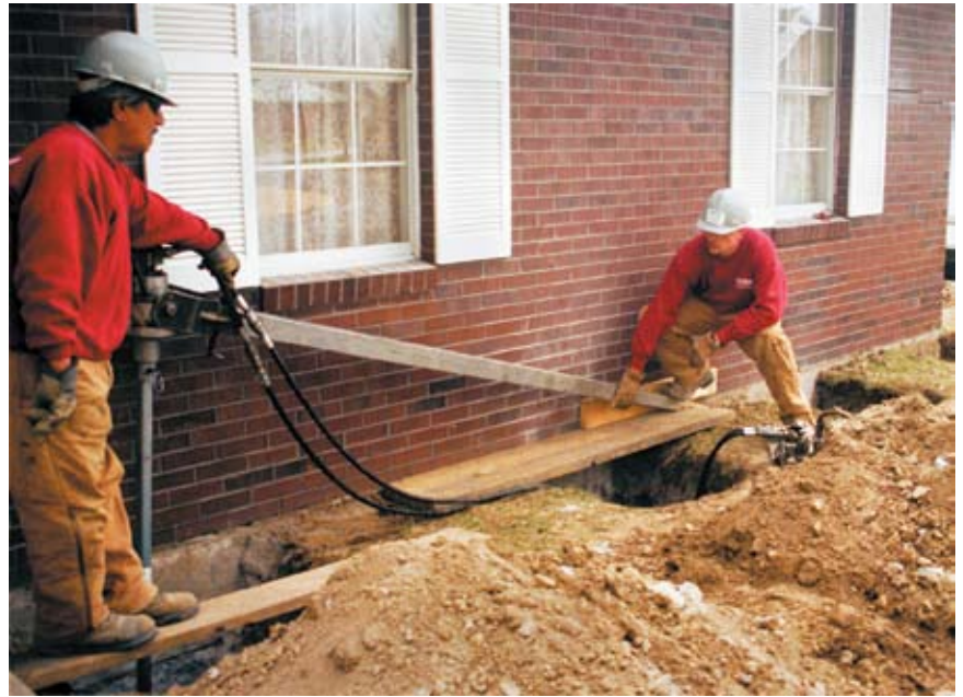
Helical pile installation by hydraulic driver
